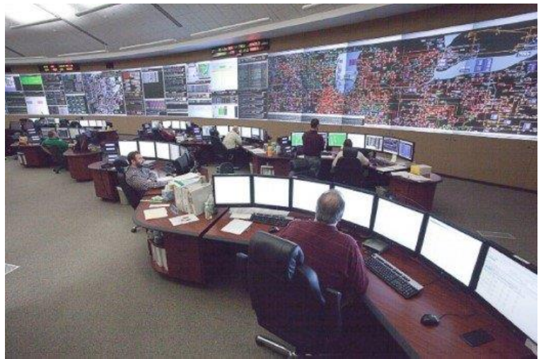
MISO control room (photo courtesy of MISO Energy)
