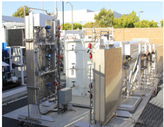
The first hydrogen fueling station in the U.S. fed directly from an active industrial hydrogen pipeline. Photo by Michael Penev, NREL 19212
